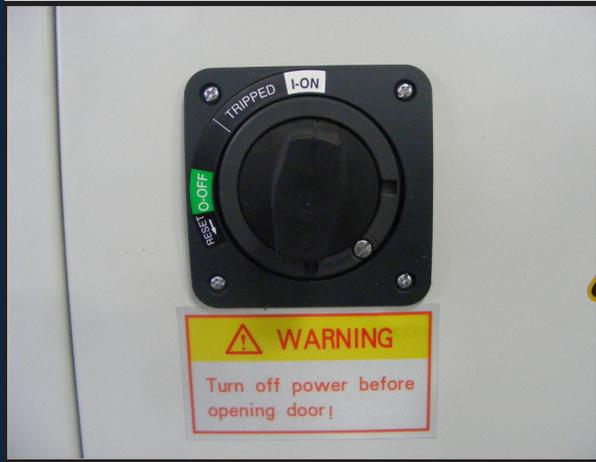
Turn the Main power switch to the ON Position.
